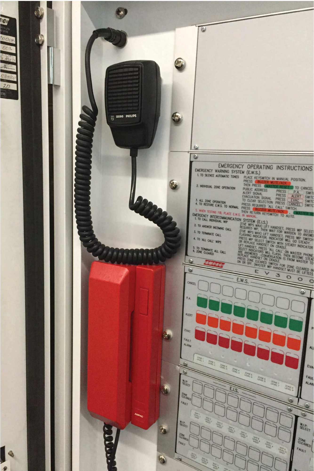
An example of good fire safety engineering, the emergency warning and intercommunication system for a 5 storey building.
