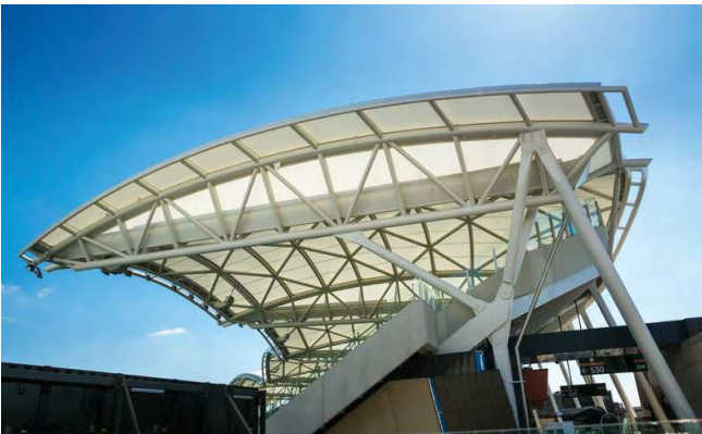
Roof over the Adelaide Oval redevelopment. Performance-Based Engineering techniques were used on the project.
